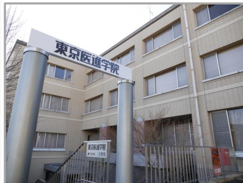
[The whole dormitory system] Mitaka School
